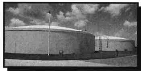
Reclaimed Water Ground Storage Tanks
