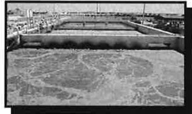
IFAS System - Aerobic AS Basin
