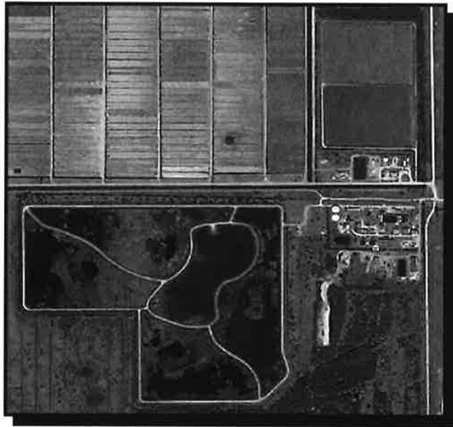
South Central Regional WRF, Wetlands and Storage Ponds
