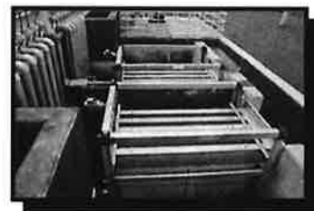
Tertiary (Disc) Filters
