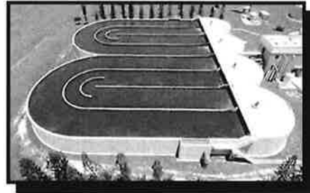
Carrousel Dual Oxidation Ditch System
