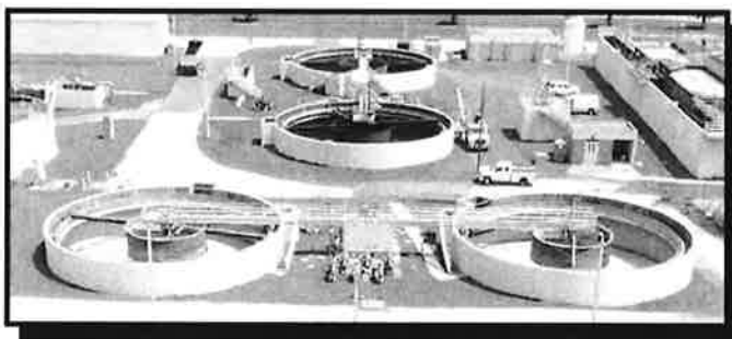
Carrousel BNR Treatment System: Sec. Clarifiers
