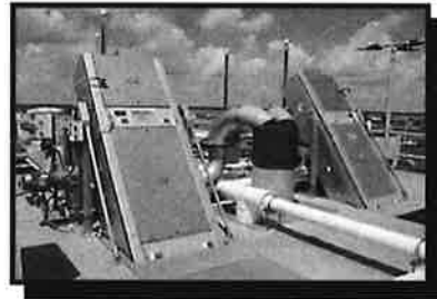
Mechanical Barscreens (3 mm)
