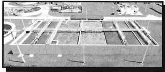
IFAS BNR Treatment System
