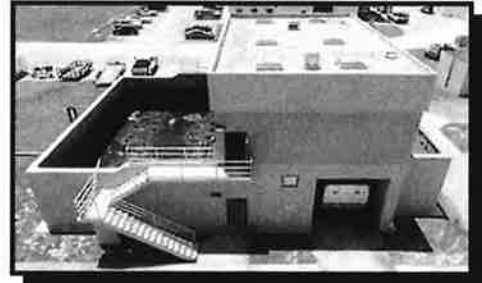
Sludge Processing Bldg/Sludge Holding Tank
