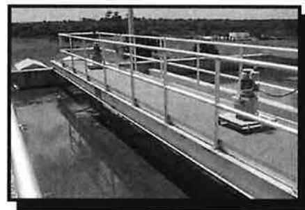
IFAS BNR System: Anaerobic Basins
