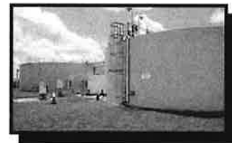
Sludge Holding Tanks
