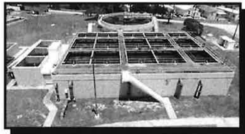
Conv. Activated Sludge Process System
