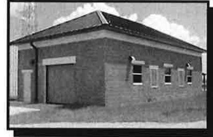
RW Distribution Pump Station Bldg
