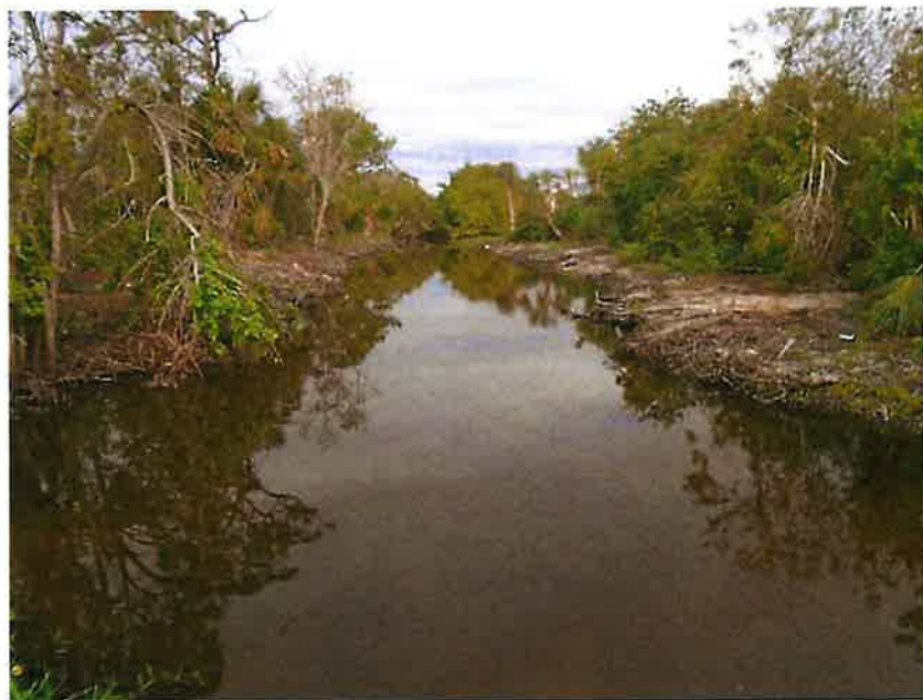
Photo 2: Photograph taken facing north into the Old Causeway Road drainage ditch. This image was taken during the inspection on December 16, 2022. Both sides of the ditch remain clear of vegetation, but some saplings of unknown species are beginning to re-establish on the eastern shore.
