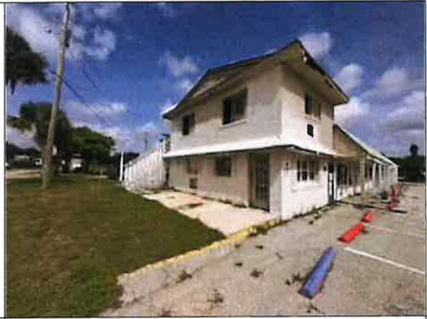
Front & Side – Southeast Corner
