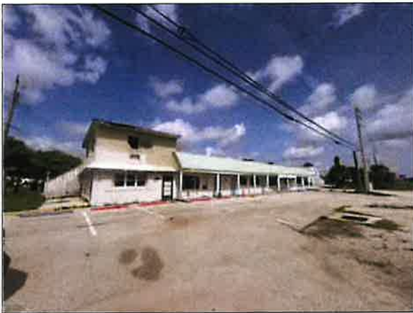
Subject Front – East Elevation
