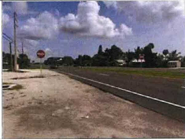
U.S. Highway 1 – Facing North
