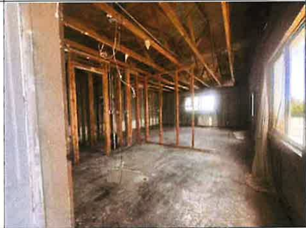
Interior of Second Floor Unit
