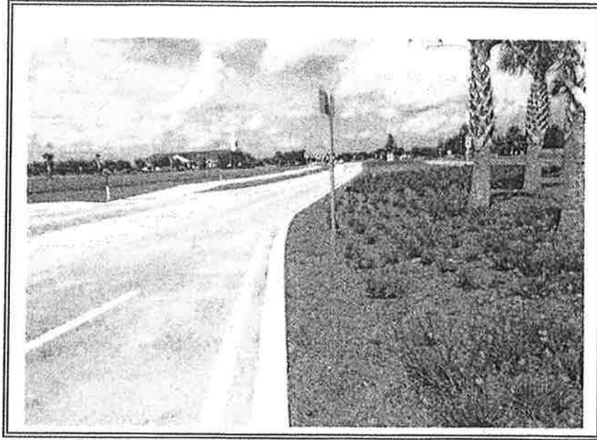
West side of center planter area
