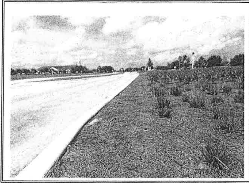
Center planter area where water is allowed to temporarily pond behind curb
