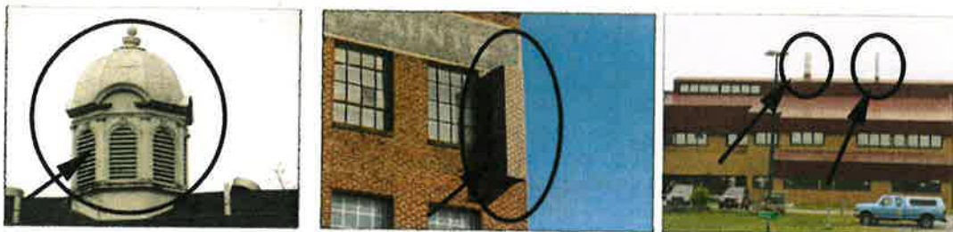
Figure 5: Examples of Antenna Concealment Techniques
