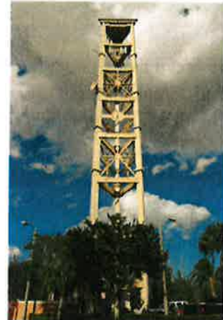
Modified Lattice Tower
