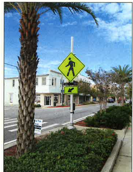
Rapid Flashing Pedestrian Warning Signals at Julia St. & Washington Ave.
