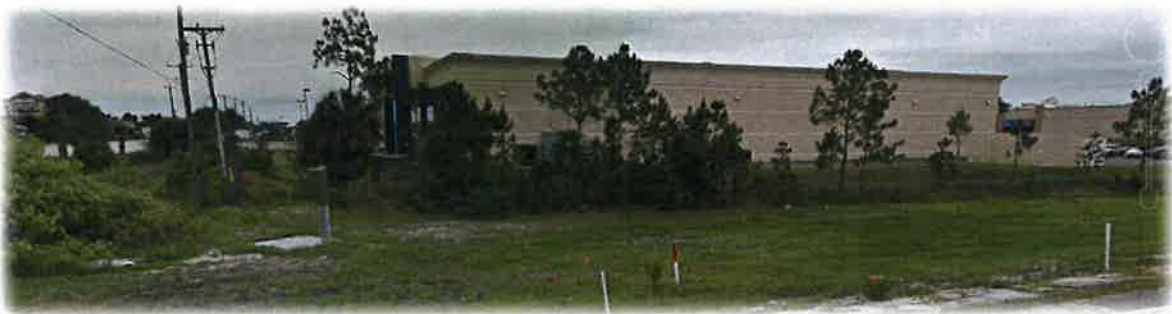
Before -Corner of New Haven Avenue and Interchange prior to landscaping
