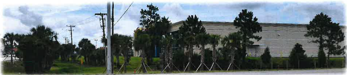
After - I-95 Landscape Improvements (FDOT grant and City of West Melbourne)
