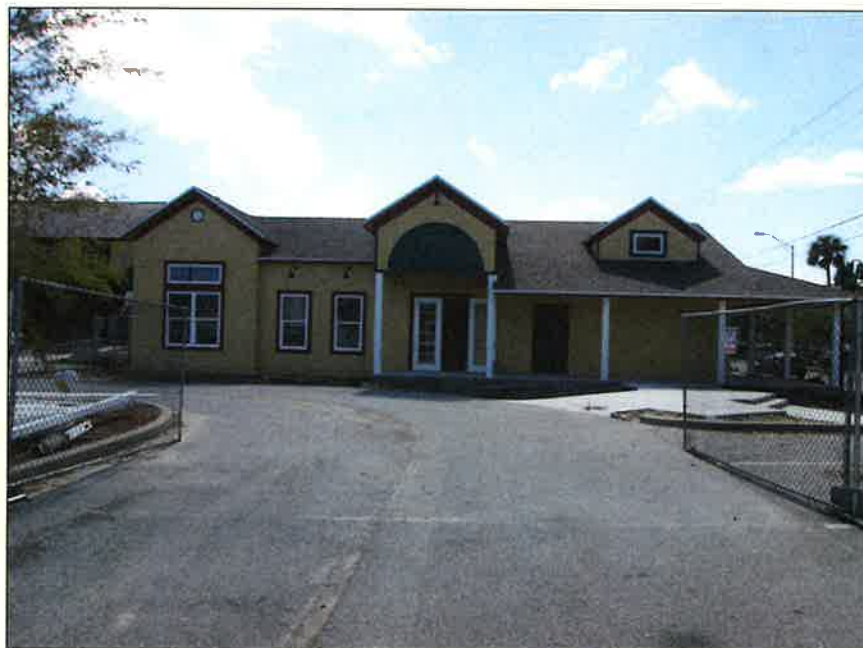
Welcome Center under construction – 9/30/16
