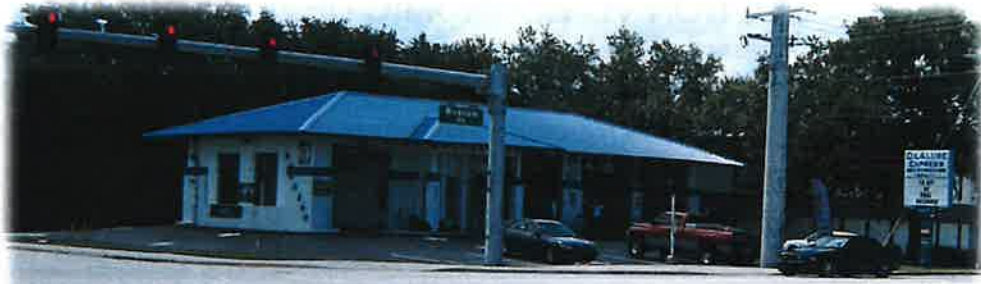
440 S. Wickham Road in 2015 before demolition
