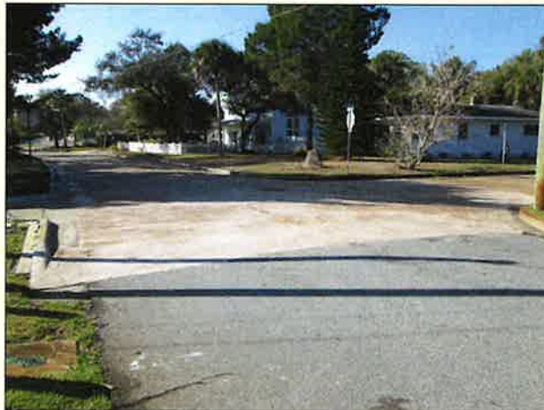
Completed concrete street repair at the Grace St. & Riverside Dr. intersection
