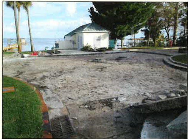
Removal and repair of concrete at the Grace St. & Riverside Dr. intersection
