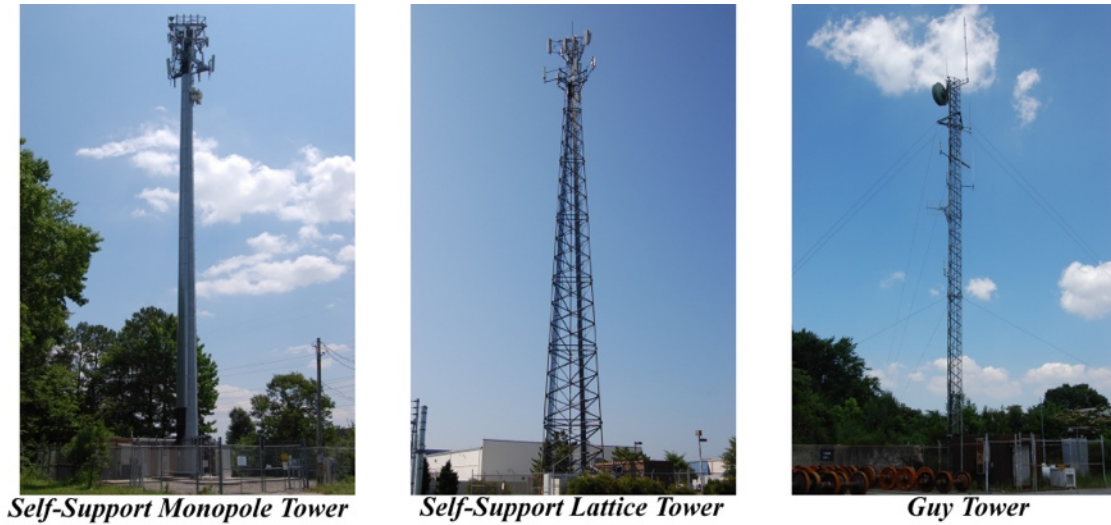
Figure 4: Examples of Non Concealed Antenna Support Facilities
