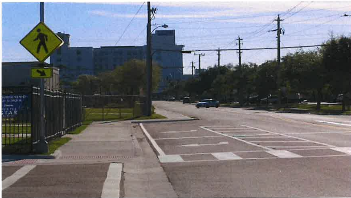
IMAGE 3- BULLDOG CONNECTION TO APOLLO WITH CROSSWALK
