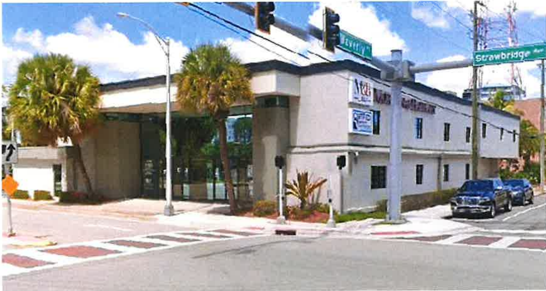
IMAGES 1-2 FAÇADE PROGRAM 730 E. STRAWBRIDGE AVENUE BEFORE AND AFTER
