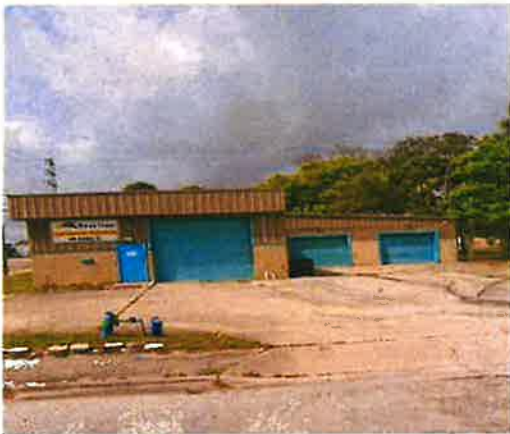
400 Garden Street Vacant Building – Before
