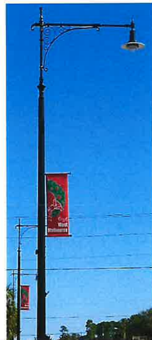
(Street lights installed in 2018 along US 192)
