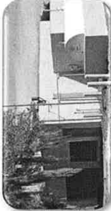
Lift Station C-18 Upgrades
