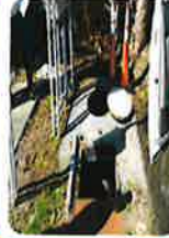
Lift Station N-3 Replacement
