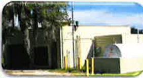
Lift Station C-18 Upgrades
