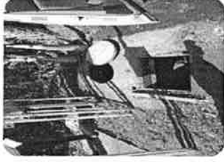
Lift Station N-3 Replacement
