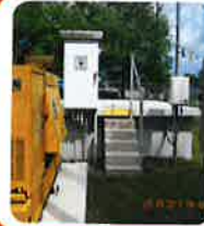
Lift Station J-02 Replacement
