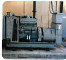
Lift Station M-20 and Generator Replacement
