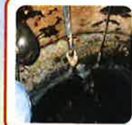
Lift Station B08 Rehab
