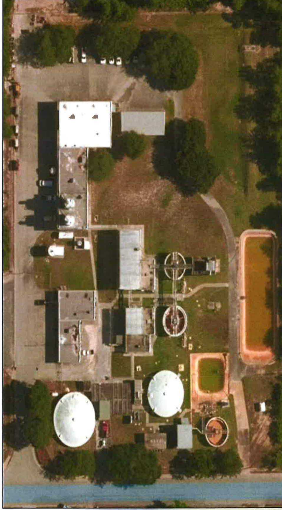
Figure 12 – Typical Water Treatment Plant
