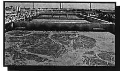
IFAS System - Aerobic AS Basin
