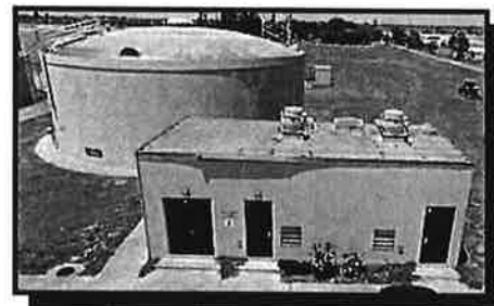
Reclaimed (Reuse) Water Pump Station
