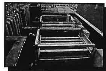
Tertiary (Disc) Filters
