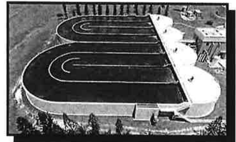
Carrousel Dual Oxidation Ditch System
