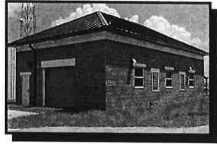
RW Distribution Pump Station Bldg
