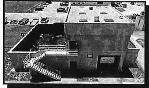
Sludge Processing Bldg/Sludge Holding Tank
