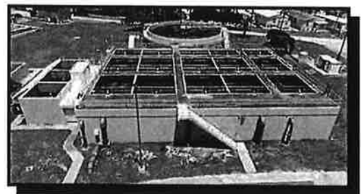
Conv. Activated Sludge Process System
