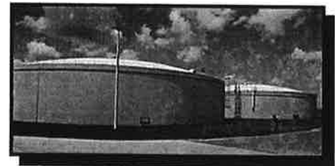
Reclaimed Water Ground Storage Tanks
