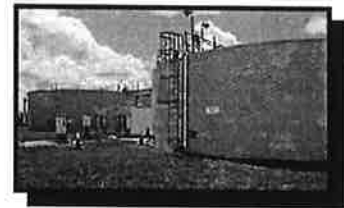
Sludge Holding Tanks
