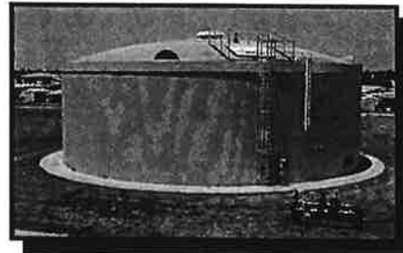
Reclaimed Water Ground Storage Tank
