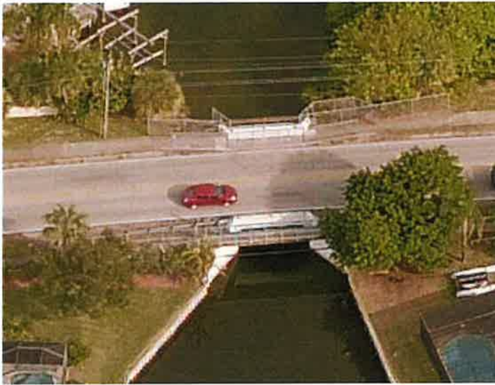
Constricted Roadway Segments over canals
