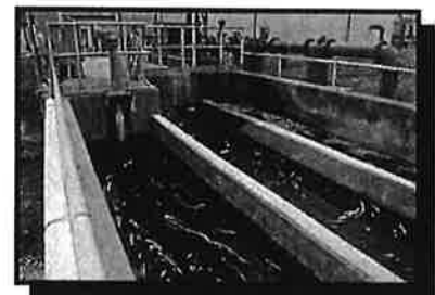
Chlorine Contact Chamber (CCC)
