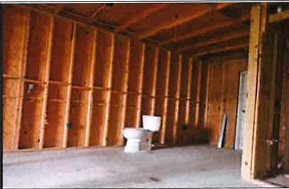
Lot 8 – Building 2 – Interior View
