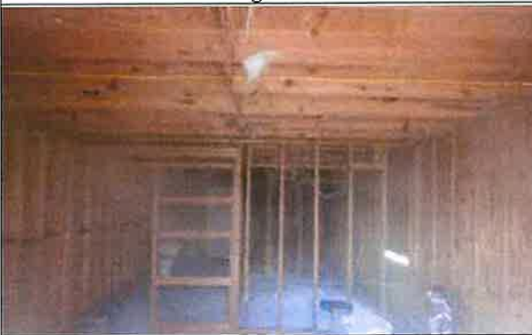
Lot 8 – Building 2 – Interior View
