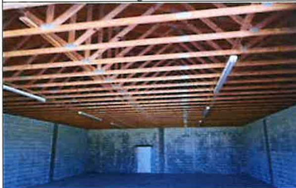
Lot 7 – Building 1 – Covered Area
