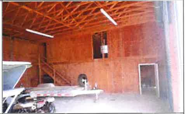
Lot 8 – Building 2 – Interior View
