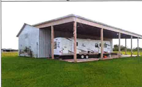
Lot 8 – Building 2 – West Elevation
