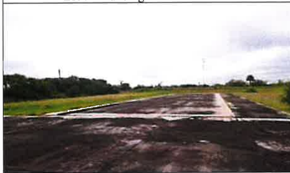
Lot 7 – Concrete Building Pad
