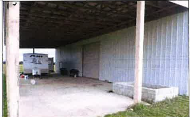
Lot 8 – Building 2 – West Elevation
