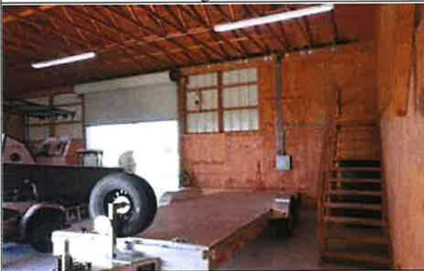
Lot 8 – Building 2 – Interior View
