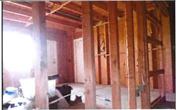
Lot 8 – Building 2 – Interior View
