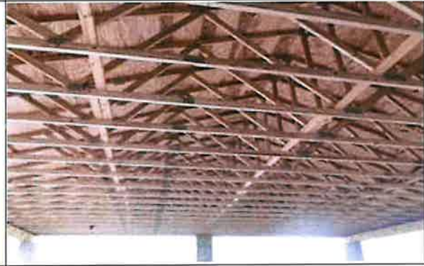
Lot 7 – Building 1 – Covered Area
