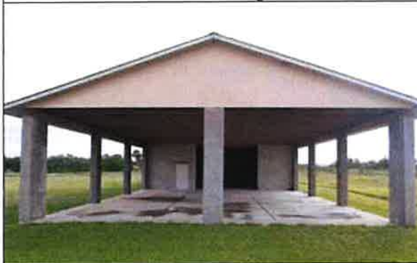
Lot 7 – Building 1 – West Elevation
