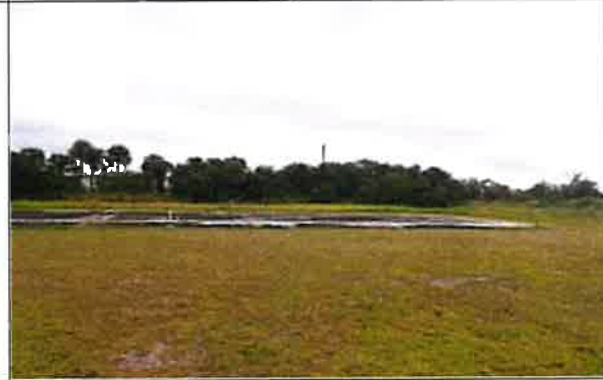
Lot 7 – Concrete Building Pad
