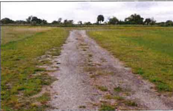
Stabilized Drive between Lots 7 and 8
