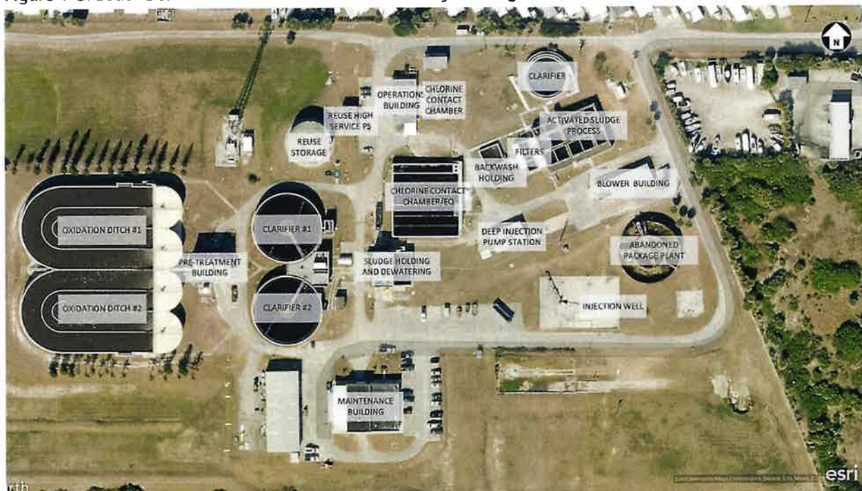
Figure 1-3. South Beaches Wastewater Treatment Facility Existing Facilities
