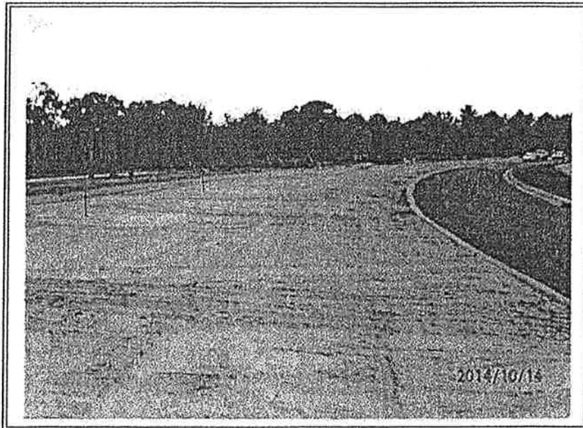
Lake Andrew Drive Phase 2A unfinished median
