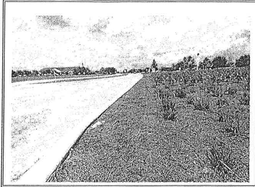
Center planter area where water is allowed to temporarily pond behind curb
