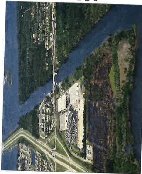
Barge Canal Area
