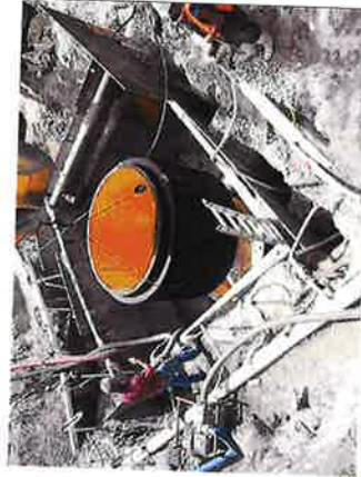
South Tropical Trail Sewer Expansion
