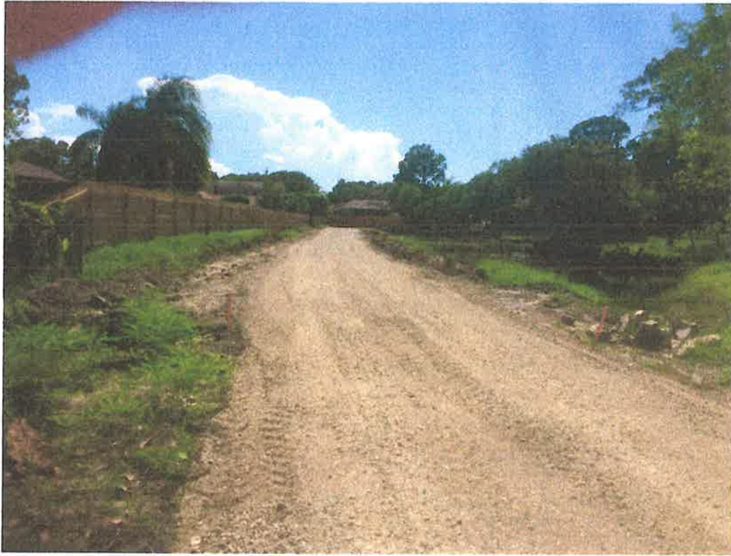
Looking West on Miller Cove Road
