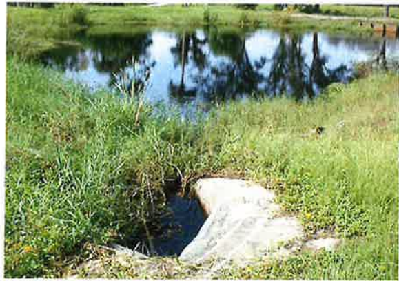
STORM BASIN FLEMING GRANT RD
