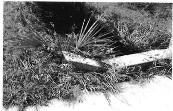
SUNK DRIVEWAY BULKHEAD
