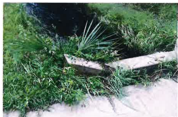
SUNK DRIVEWAY BULKHEAD
