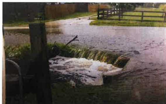
STORM RUN OFF
