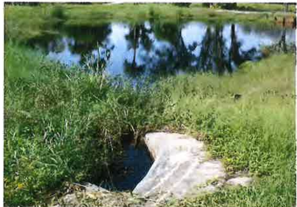
STORM BASIN FLEMING GRANT RD
