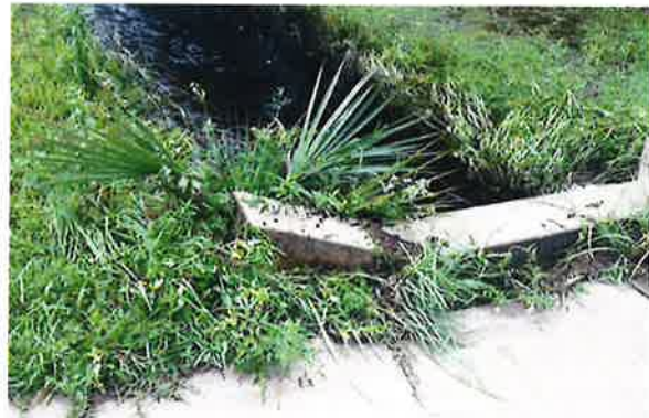
SUNK DRIVEWAY BULKHEAD
