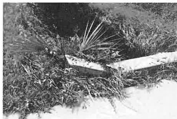
SUNK DRIVEWAY BULKHEAD
