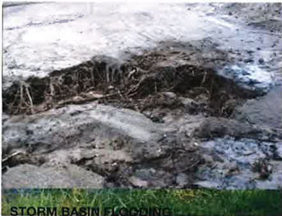
STORM BASIN FLOODING
