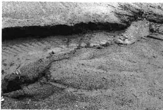
STORM BASIN FLOODING
