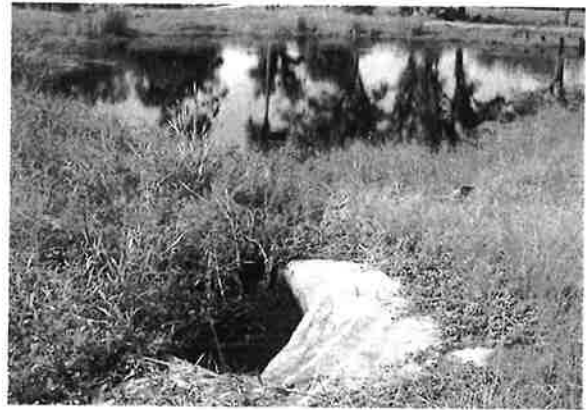
STORM BASIN FLEMING GRANT RD
