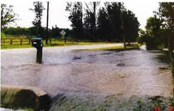
STORM RUN OFF
