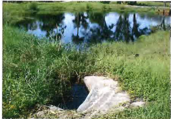
STORM BASIN FLEMING GRANT RD
