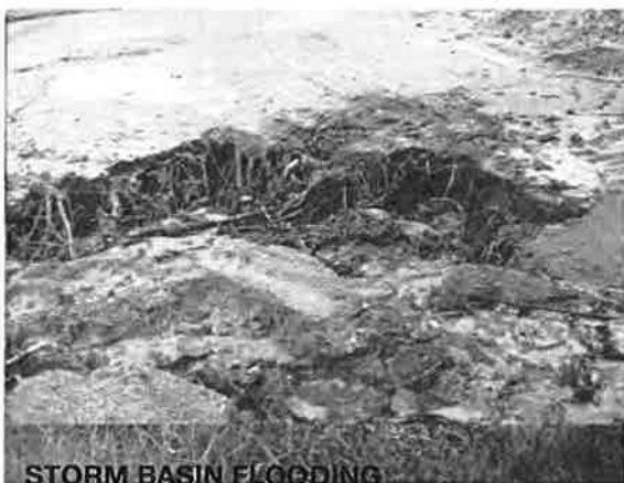
STORM BASIN FLEMING GRANT RD
