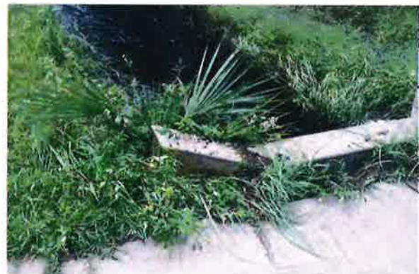
SUNK DRIVEWAY BULKHEAD
