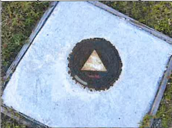
Well Cap on Parcel D
